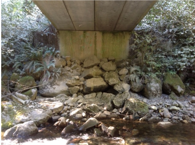
Right Bank Abutment when facing downstream
