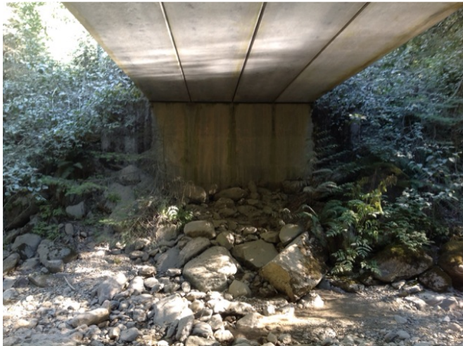
Left Bank Abutment when facing downstream
